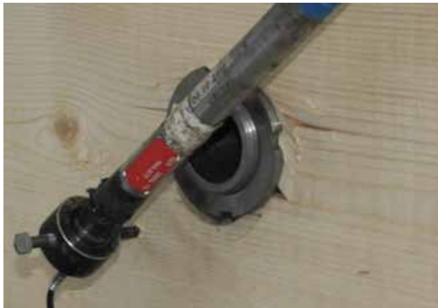
Figure 9. Deformation of central joint in the second truss
