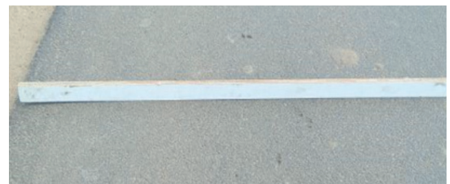
Figure 5. Newly constructed road surface on January 2015
