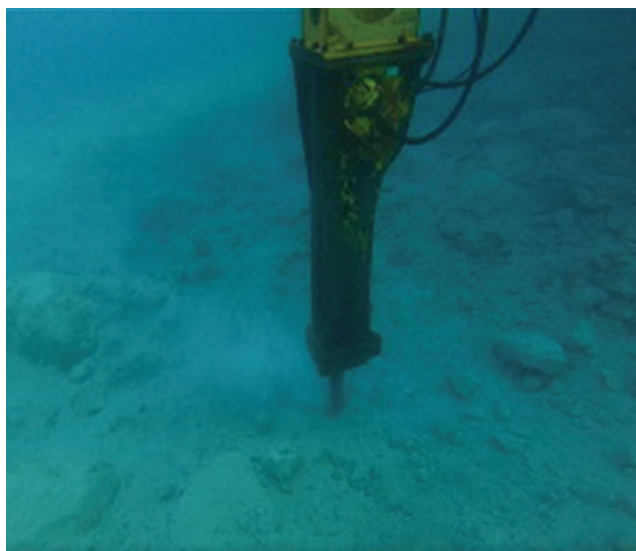
Figure 12. Excavation using a pneumatic hammer [28]
