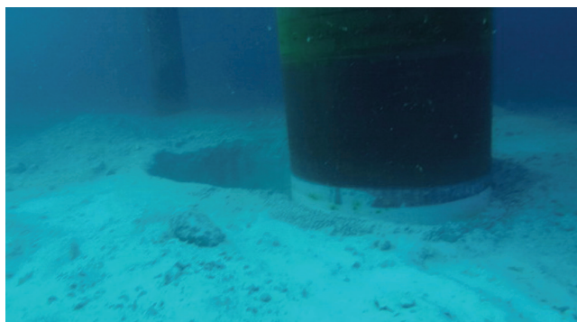
Figure 10. Excavation using a drill [28]
