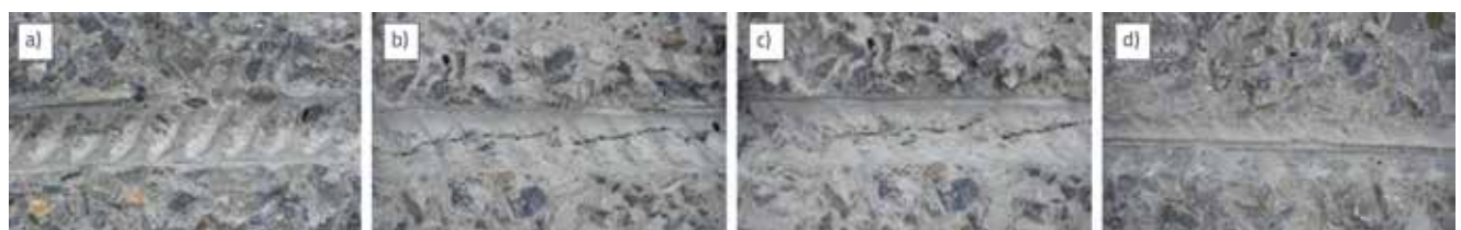
Figure 8. Damage photos of internal bonding surface after microwave irradiation: a) 0 W; b) 1000 W; c) 3000 W; d) 5000 W
