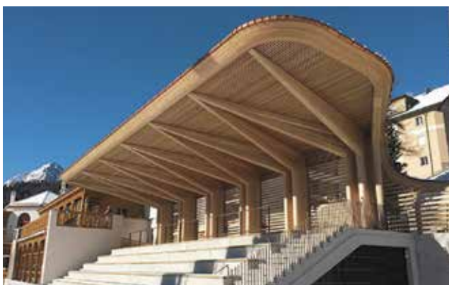
Figure 1. GLT made of ash wood – Grandstand of Kulm Hotel in St. Moritz [5]
