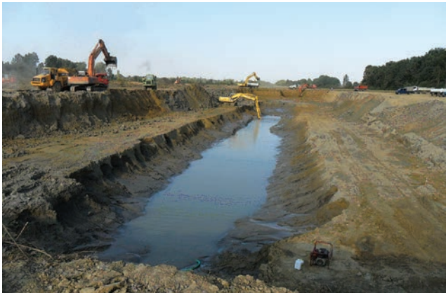
Figure 6. Canal excavation works [13]
