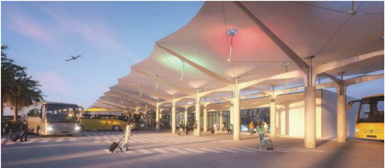
Figure 21. New shed in front of the bus terminal building
